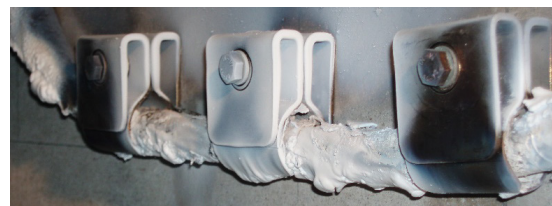
Phoenix clips have been fire tested in accordance with BS 5839-1: 2017.
