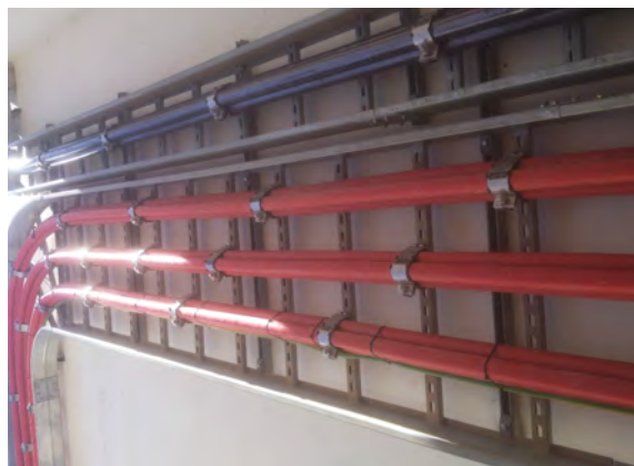
THE LATERAL LOAD RATING OF A CLEAT CAN BE USED TO SPECIFY CLEATS BASED ON CONTINUOUS LOADING, SUCH AS MOUNTING CLEATS ON A SIDE.
